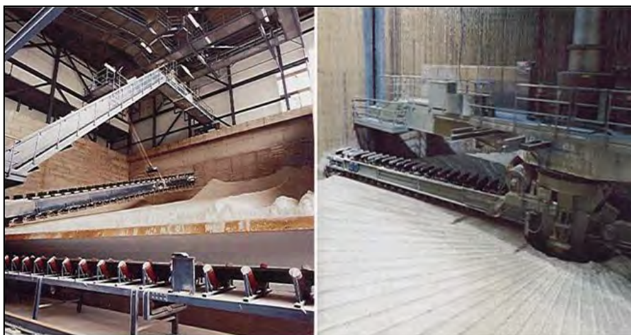
Figure 4.23: Closed gypsum storage facilities [94, Umwelt + Technik, 2000]
